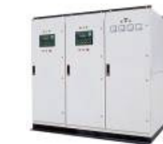
DSE-550 Parallel Control Panel system
